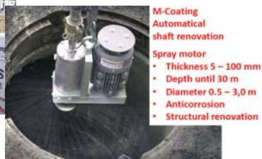
M-Coating ready to begin after cleaning with the TSSR
