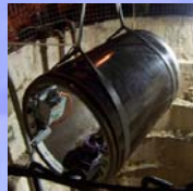
jacking pipe with equipment for online load control system
