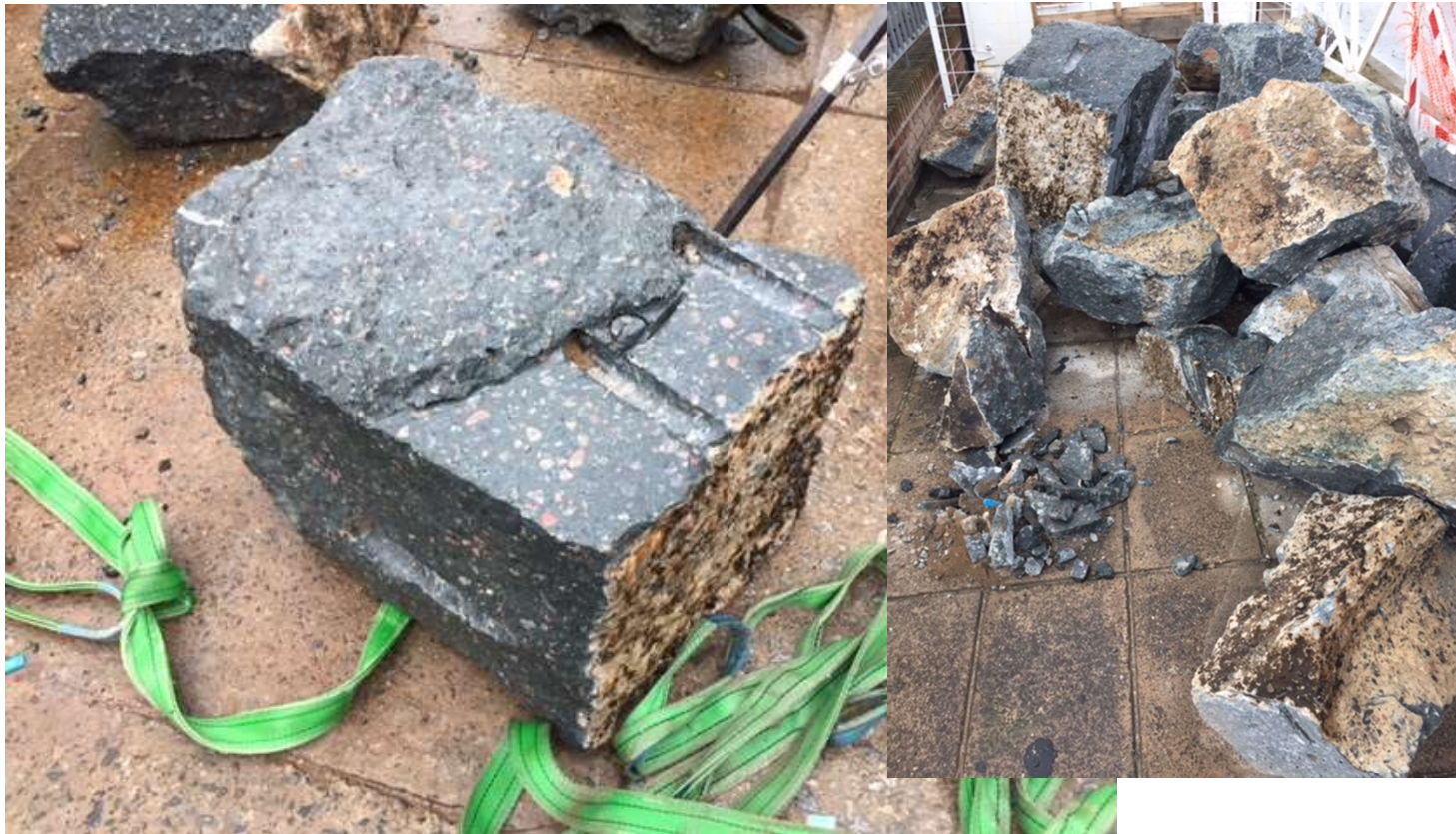
Expansion of concrete sedimentation by diamond saws an hydraulic splitter
